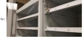
3.9. To access the cabinet **drawers**, unlock the two camlocks, 8001 on the front-left, 8011 on the right of the cover in this order. You cannot remove 8011 until the cover is open.
